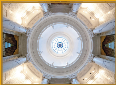
Interior view of the Legislative Library's central dome. The eight massive columns supporting the dome are made of scagliola – a decorative form of plaster that is molded and hand-painted to imitate marble.
